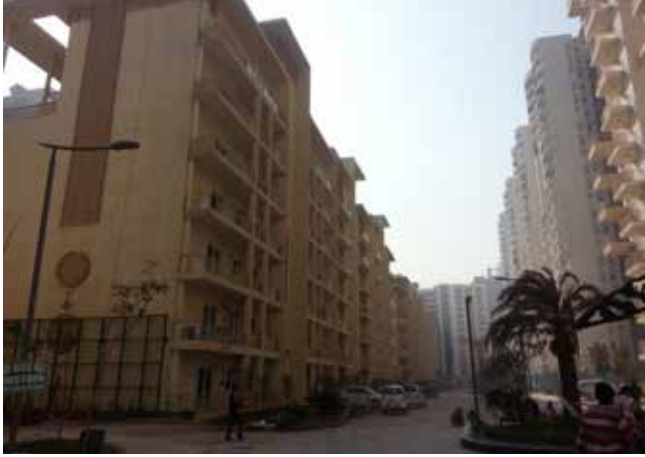
Low Rise Towers
